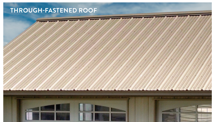
83 screws per 100 sq. ft. (exposed)
